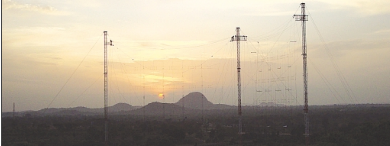
Bodo, DL3OCH, used this impressive curtain array of 16 dipoles as 5N00CH during the contest. This antenna will be used for commercial broadcasting once it is put into service.
