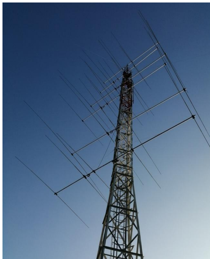
9A7A Tower #2 holds a stack of 3 x EF204ARC antennas for 20 meters and a stack of 3 x EF155C antennas for 15 meters. These antennas are also of YU7EF design
