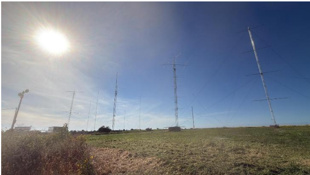
I19P Antenna Farm – I19P Multi-Distributed
