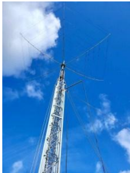
Temporary antenna installed at G2EC - G3TXQ Hexbeam on Versatower P60
